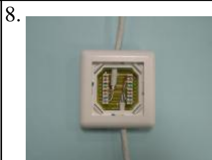
Put frame on base housing again.
