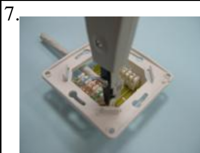
Use a punch down tool to complete the termination and cut off any access wire.
