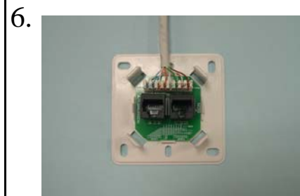
Follow the direction on the color coding to position T568B or T568A wiring, separate a little space on proper position and insert the 4 pair wires into the slot, then keep the twist as near IDC as possible.
